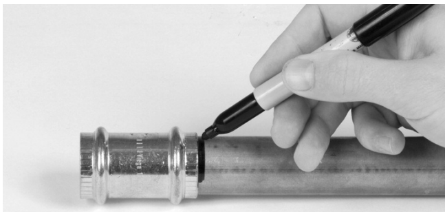
Figure 8 – Marking the Tubing After Fully Inserting Tube
