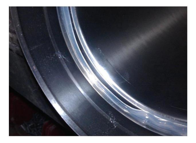
2. Smooth the bead of silicone down with your finger to spread. Remove any excess caulking.
