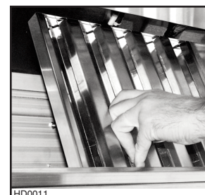
BAFFLE FILTER (TYPICAL)
