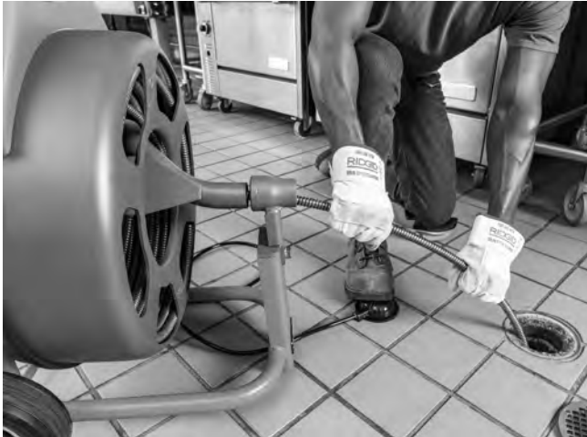
Figure 12 – Feeding of the Cable
