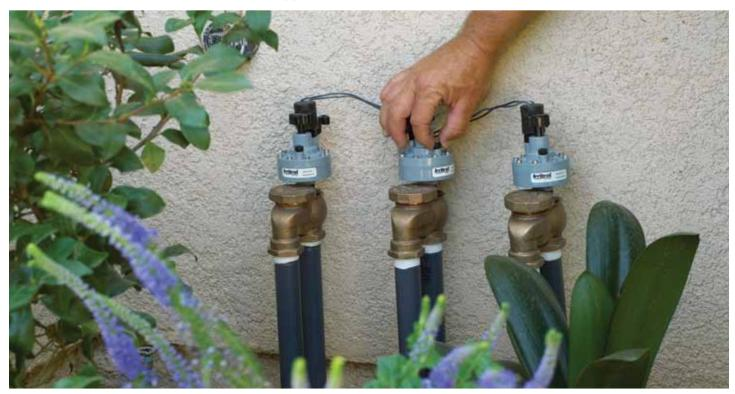
These electric anti-siphon valve adapters feature outstanding durability for consistent, dependable performance in all types of applications. Plus, having all of the internal components captured in a single unit means converting manual valves to electric doesn't get any easier.
