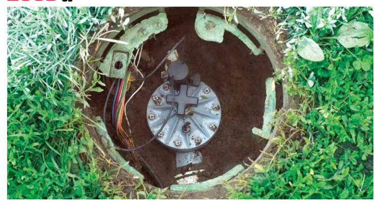
The Irritrol® 200B Series globe/angle valves have built their popularity on a proven record of reliability and a reputation for offering valuable features at an affordable price. The 200B Series provides manual internal and external bleed, heavy-duty, UV-resistant PVC construction, stainless steel hardware, a double-beaded diaphragm and a captive solenoid plunger.
