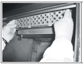
**2.** Once you remove the flame shield, you'll find the combustor. The honeycomb combustor can be made of different materials such as cordierite, mulite or even stainless steel. They are all the same with regard to removal and caution should be taken so as to not drop or damage the combustor. If your combustor has never been cleaned according the manufacturers directions, you may wish to clean the combustor before replacing it with a new combustor, see "CATALYTIC COMBUSTOR CLEANING" on page 26.
